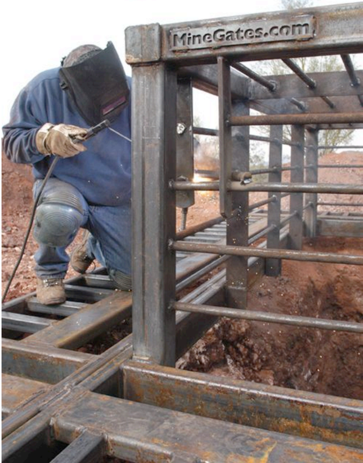
Final Cupola Bat Gate Welding
