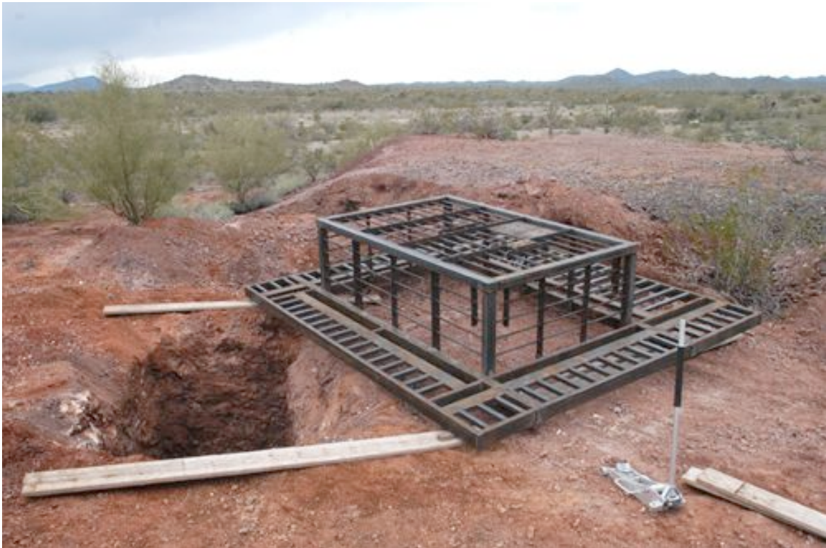
Placing Cupola Gate over the Mine Shaft
