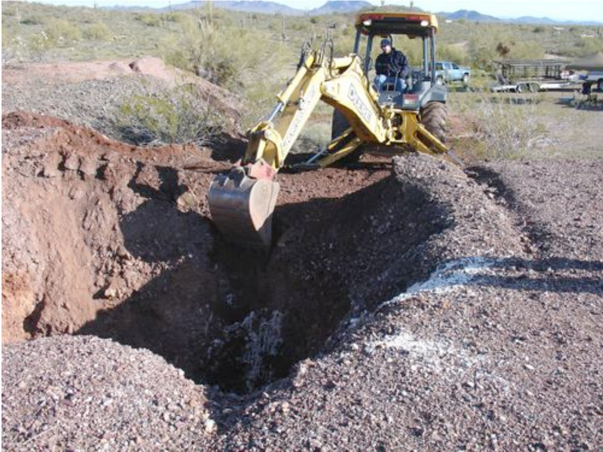
Careful Backhoe Clearing of Waste Rock Around Mine Shaft Collar
