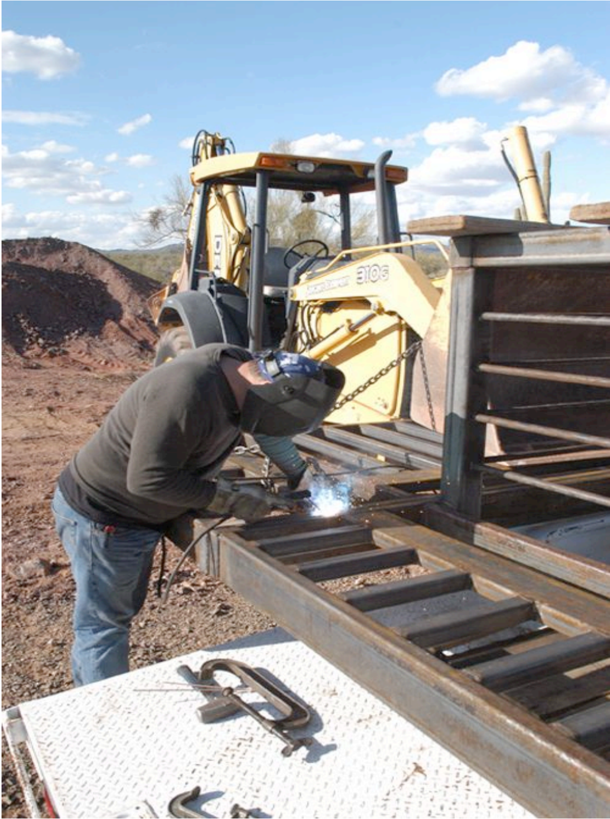
Welding Stability Apron to Main Cuploa Bat Gate
