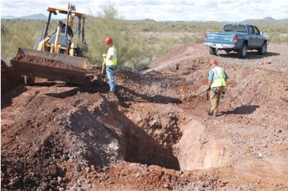
Backhoe and Hand Clearing of Waste Rock Around Mine Shaft Collar
