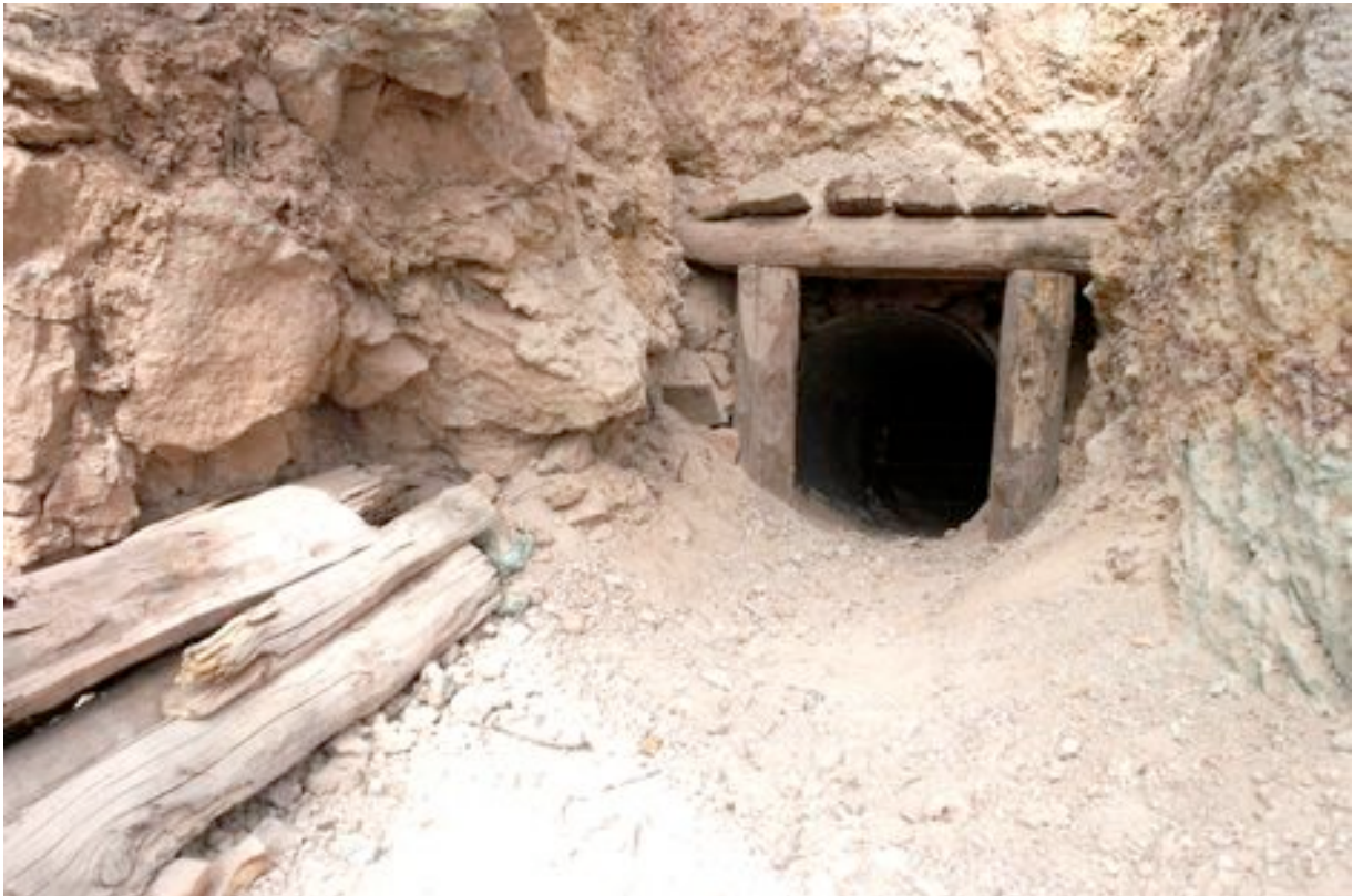
Culvert Gate with Historic Shoring Timbers
