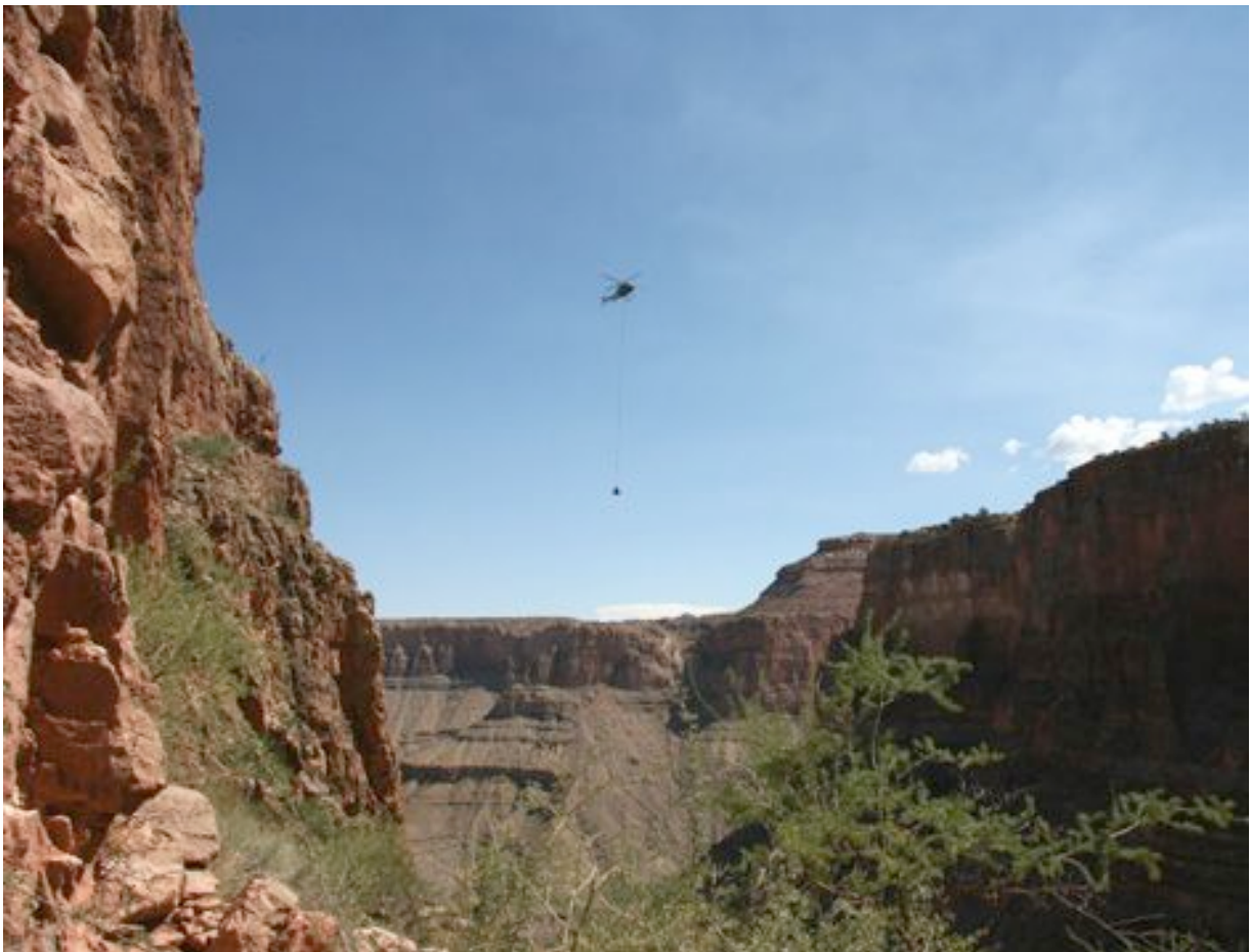
Helicopter Hauling Equipment to Last Chance Adit
